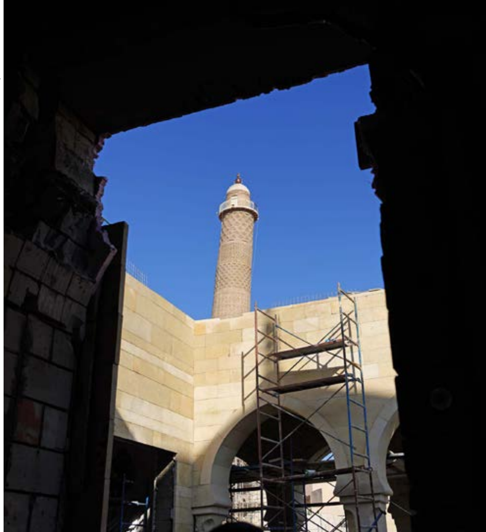
▼ Reconstructing the leaning Al-Hadba minaret.
