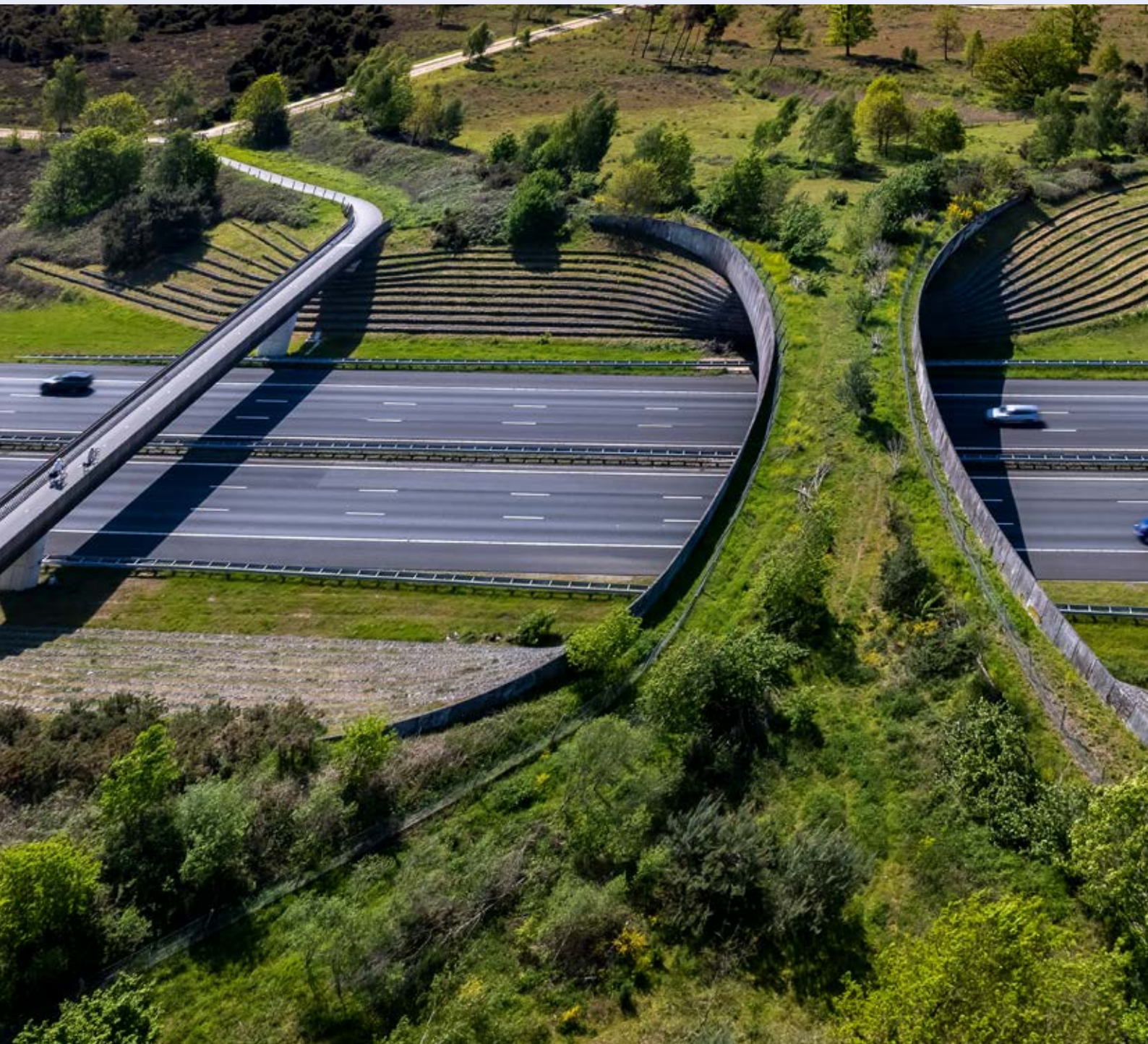
▼ The De Borkeld ecoduct in the Netherlands.
